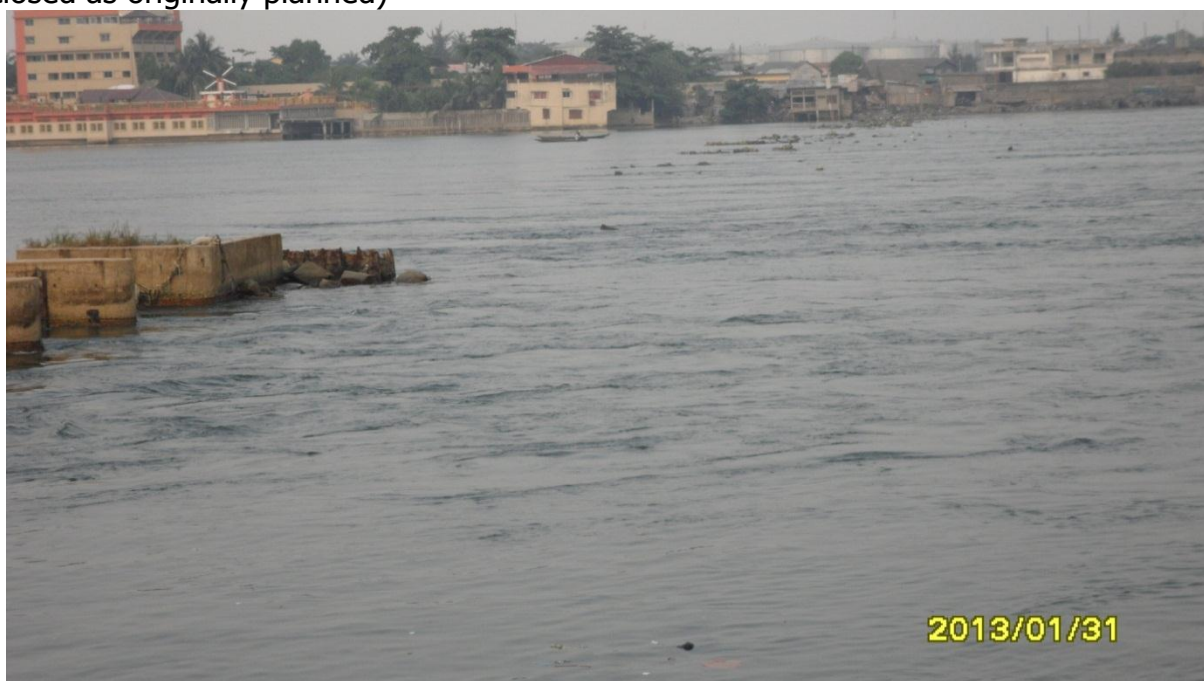
PHOTOGRAPH No. 07: The dam is entirely flooded during half tide.
