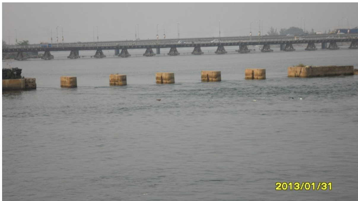
PHOTOGRAPH No.06: Here are the lagoon dam channels (there have never been closed as originally planned)
