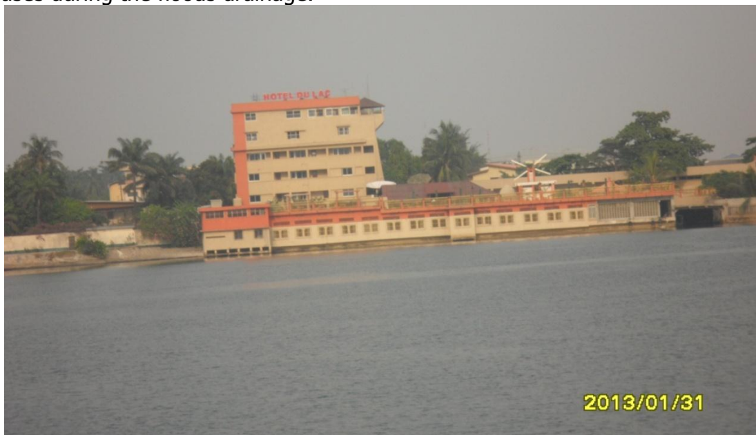
PHOTOGRAPH N°08: The Hôtel du lac alongside the lagoon between the old bridge and the dam
