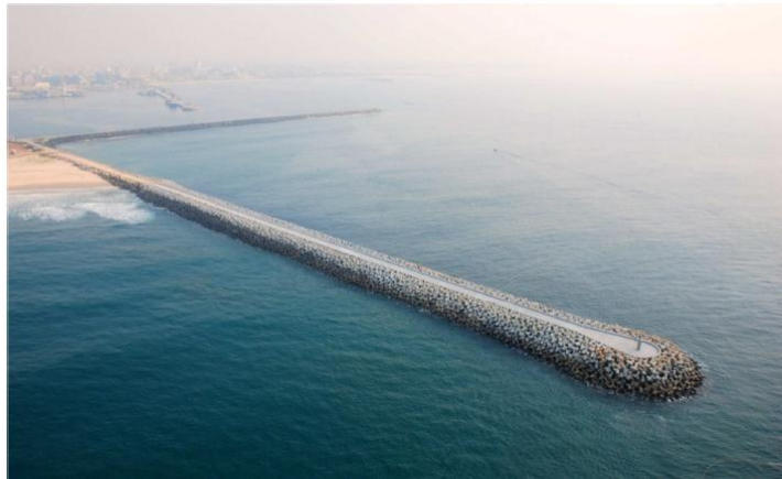
Figure 1.12 : Sand stoppage groyne at the Cotonou sea port extended to 300 in 2010.
