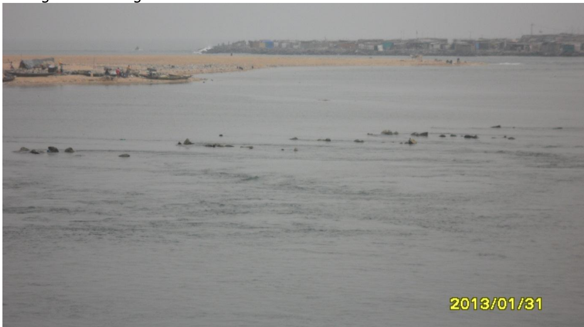
PHOTOGRAPH No.01: view of the west breakwater, the sand arrow and part of the dam
