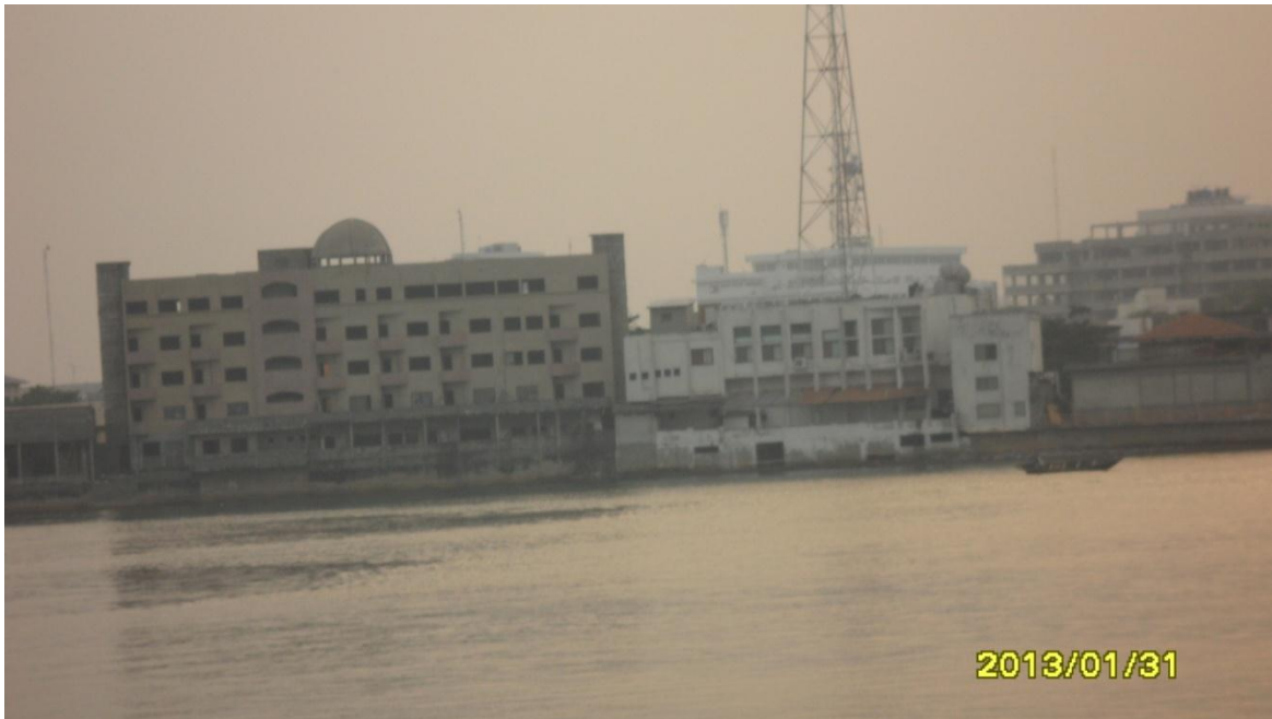
PHOTOGRAPH No.11 : Other tourist facilities alongside the lagoon between the bridge and the dam.
