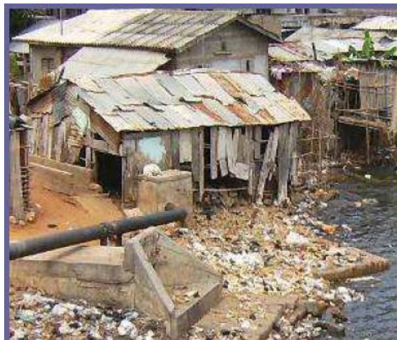
Figure 2.1 : Outlet of rain waters or waste waters’ main sewer, drink water conduits stripped by erosion in an unhealthy environment on the banks of the Cotonou lagoon
