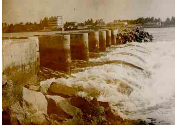
Figure 25 : Slides gates Dam at the mouth Cotonou channel
