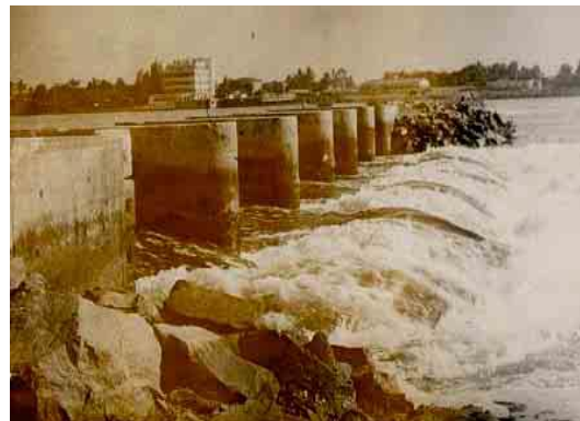
Figure 2.4 : Dam with gates at Cotonou Lagoon outlet
