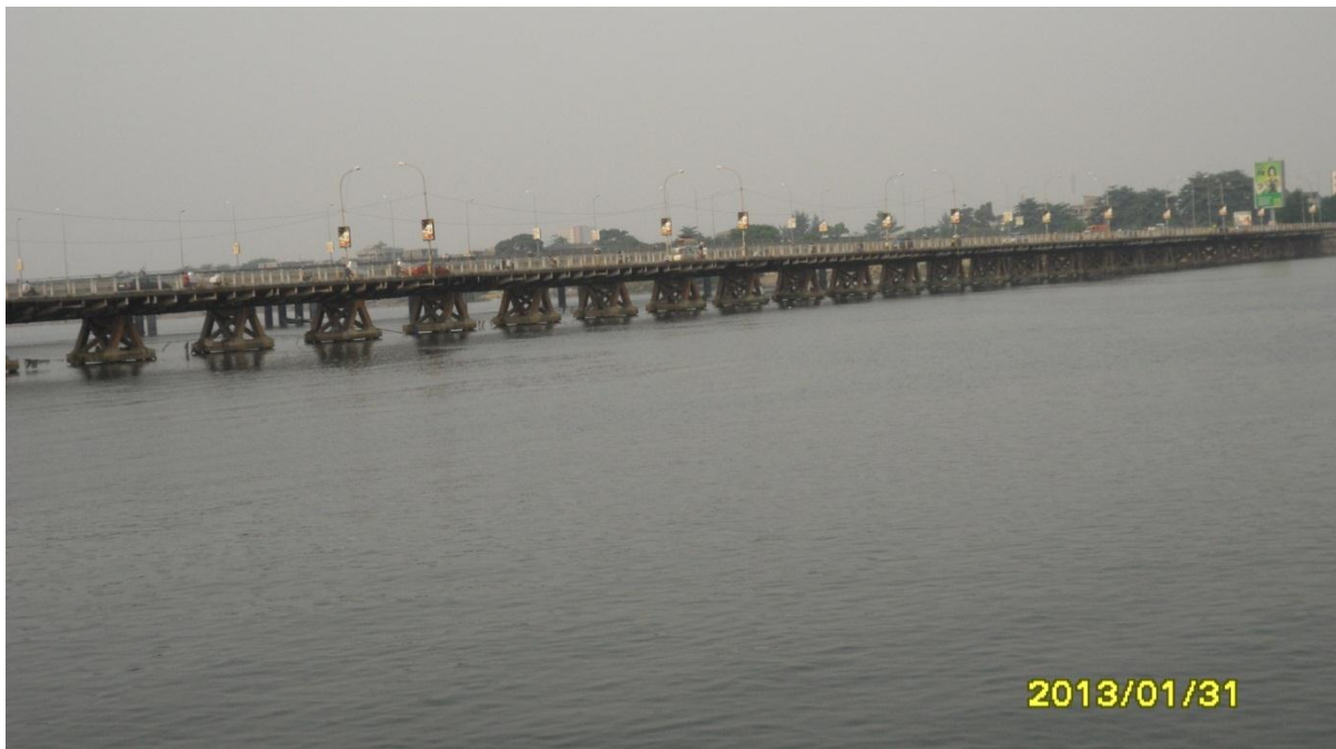
PHOTOGRAPH No. 08: The Cotonou lagoon first dam foundations which were threatened by the erosion of the bottom of the lagoon outlet
