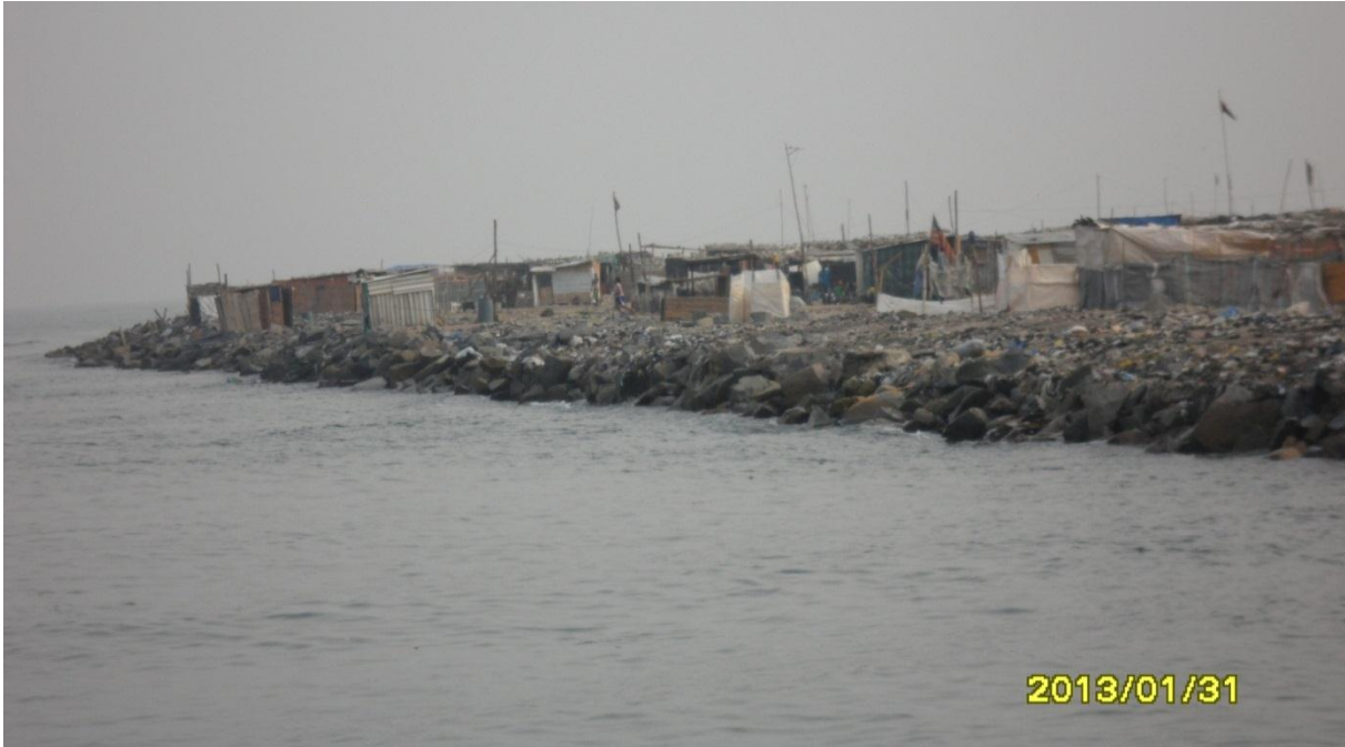
PHOTOGRAPH No.3: The western lagoon shore longitudinal protection at a point located between the western breakwater and the breakwater in the lagoon
