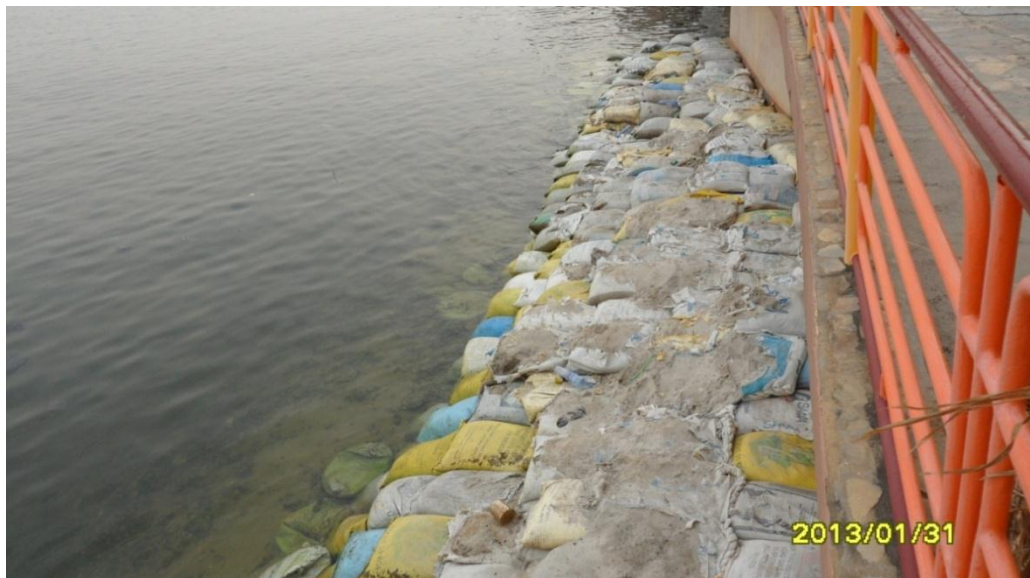
PHOTOGRAPH No.9: Protection of the front floor of a restaurant alongside the lagoon (the Restaurant Berlin)
